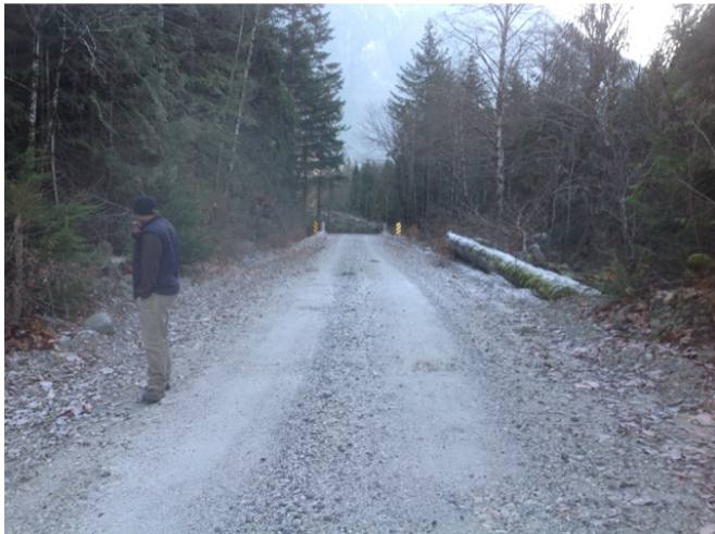
Approach from Right Bank when facing downstream
